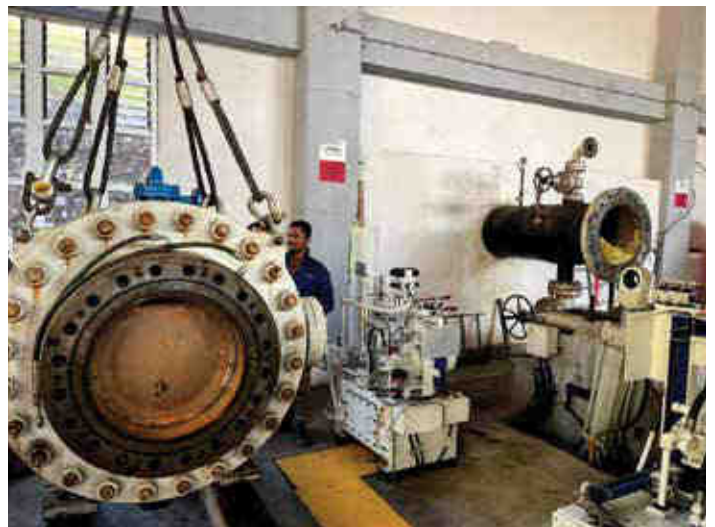
▶ Maintenance of Spherical Valve
