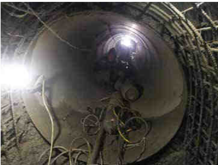
▶ Pipe Insertion for Tunnel Repair
