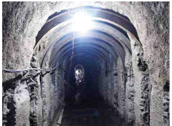
▶ Repair of Tunnel
