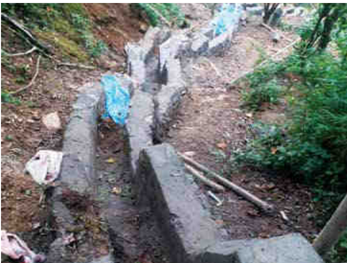
▶ Construction of Drainage
