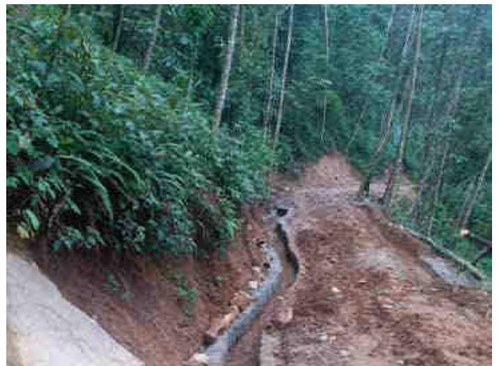
▶ Construction of Drain
