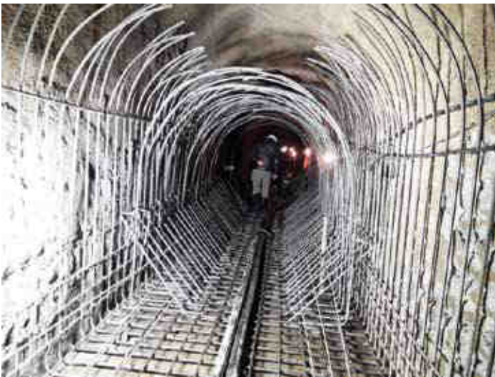
▶ Repair of Tunnel
